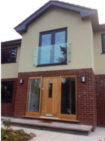
This is a guide which should help when installing a glass Juliette balcony into masonry using threaded bar and resin (also known as chemical fixing). We supply a 17.52mm toughened laminated glass panel with either 4 or 6 nr stainless steel glass adaptors (generally anything above 1.5m will have 6). The adaptors have an M10x300mm thread. This can be unscrewed, if required.
